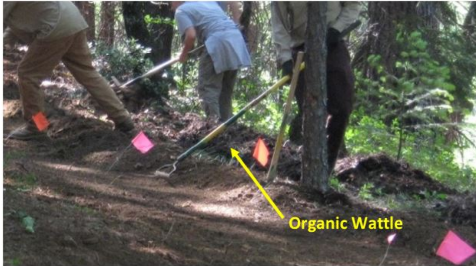
Photo 27.2 - Raking Organic Material Below the Trail to Form a Wattle
