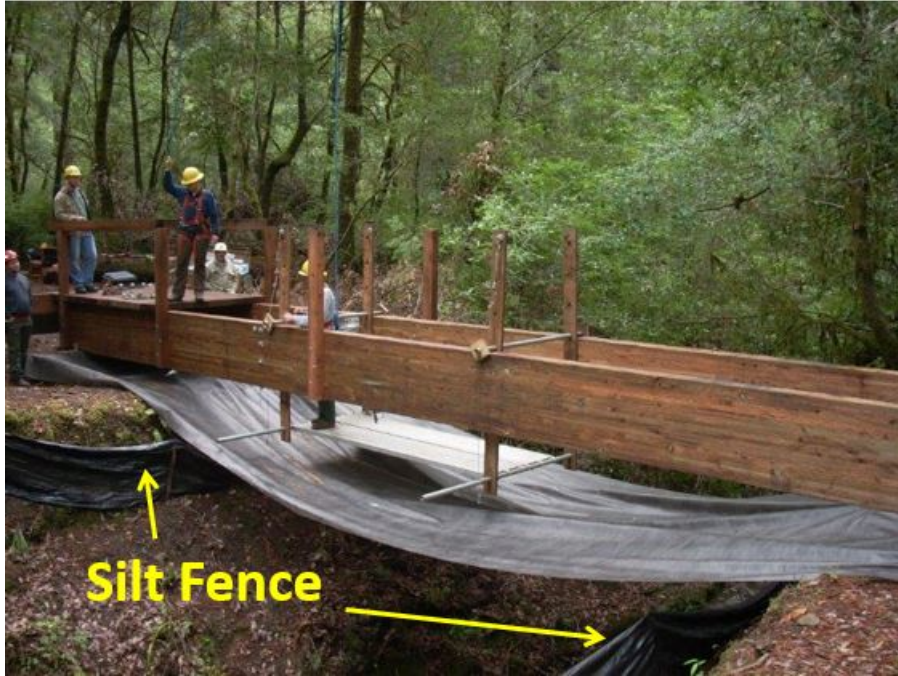
Photo 27.4 - Silt Fences Installed Between Bridge Abutments and Stream Channel
