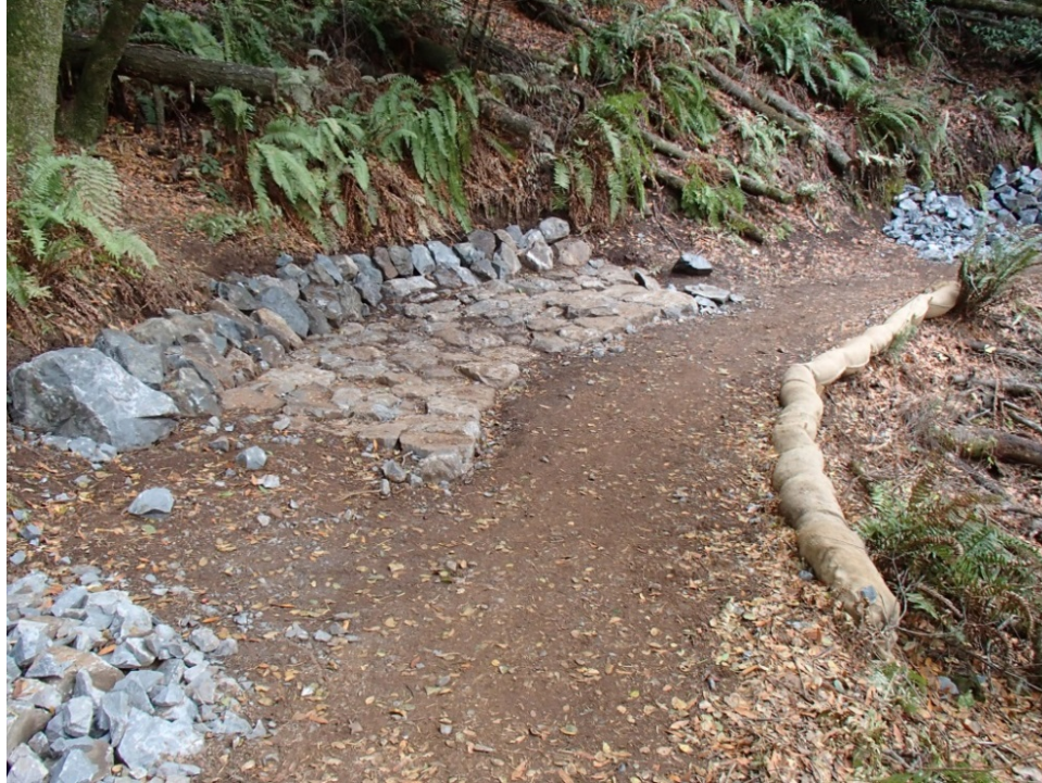
Photo 27.6 - Straw Wattle Installed Below Work Area for Construction of Armored Swale
