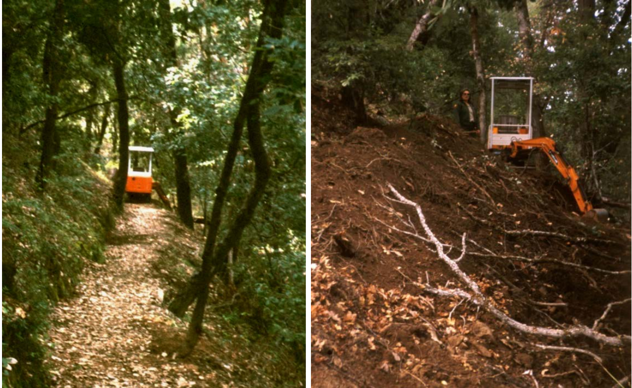
Photo 27.7 - Mini Excavator Recontouring a Trail Prism
