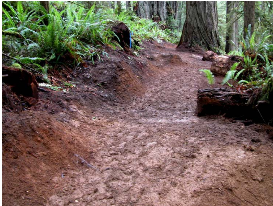
Photo 27.1 - Tread Excavation When Soil is Very Wet
